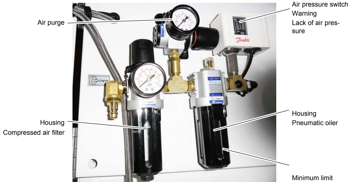
Img. 10-3: Compressed air service unit
